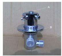
2 Lift up wall plate (B) to expose temperature indicator band, mark band to body thread position with maker pen as (C) Now undo the head by unscrewing the phillips retaining screw inside the cap aperture A.
